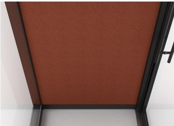
The interior side fascias are composed of acoustic tackable fabric, providing sound absorption, a place to pin notes and a soft, comfortable visual aesthetic.
